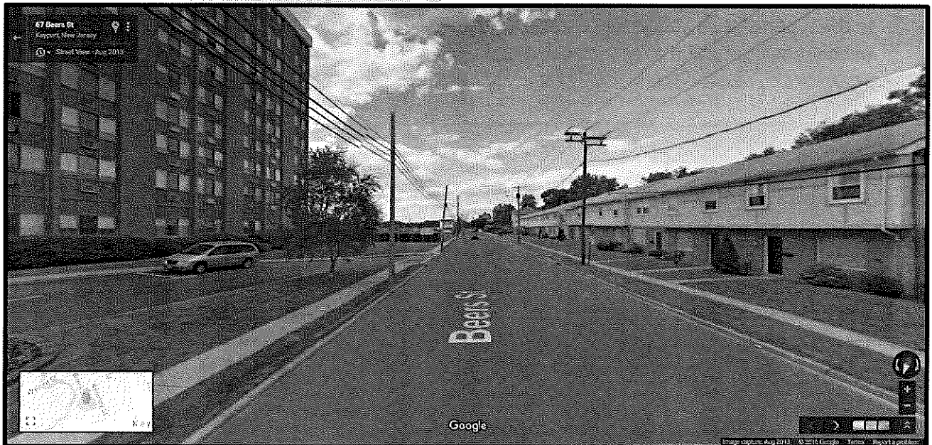
Figure 24 View of Beers Street overall width
